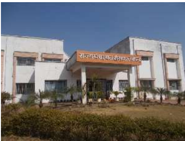
Main Building of SIRD Complex
