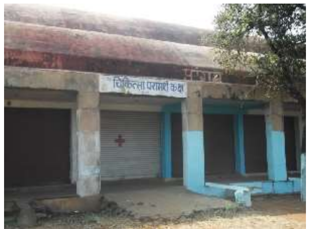
FACILITIES WITHIN WALMI COMPLEX
