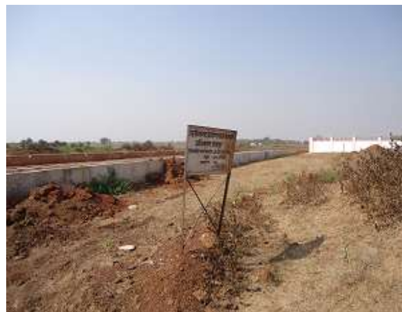
Site for RRNMU – Sector-24, Naya Raipur
