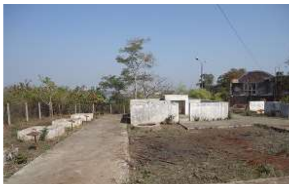
Structures of Sanitation Demonstration Project
