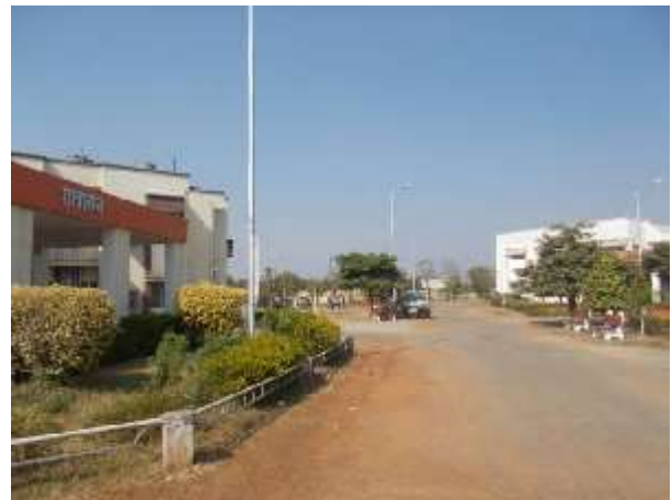
Existing Hostel within SIRD Complex
