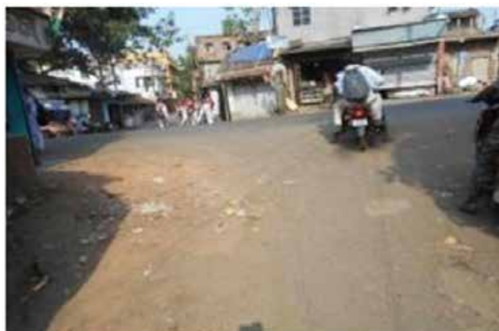
a) Vertical Alignment not Levelled
