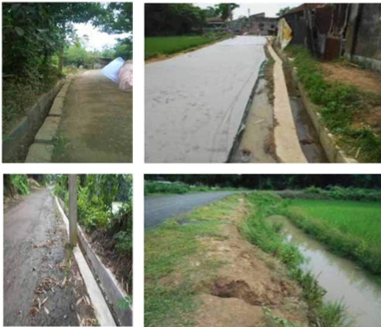
Figure 3-9: Road Side Drains
