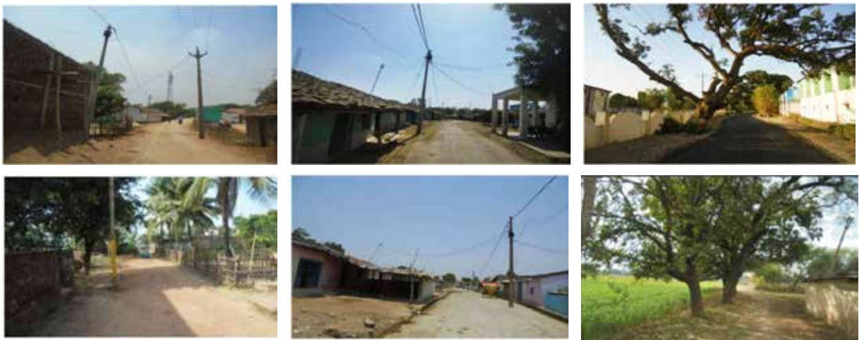
Figure 3-8: Road Side Hazards (Trees and Poles on/close to Carriageway)
