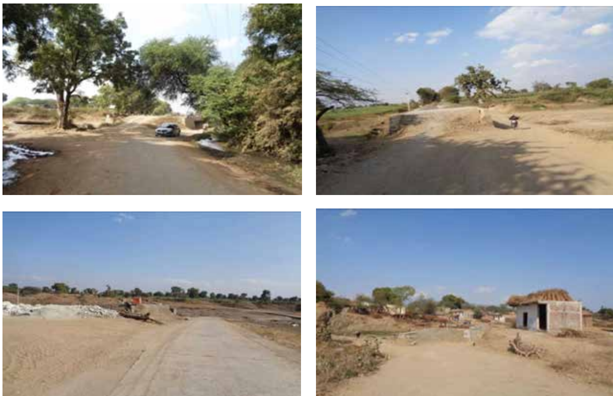
Figure 3-10: Unsafe Work Zones
