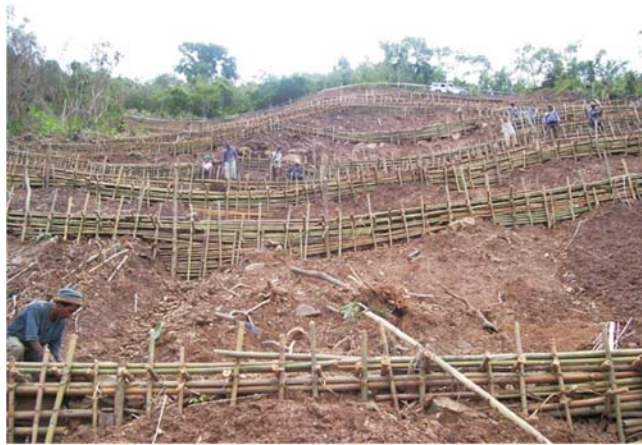
Bamboo Crib wall built by villagers
