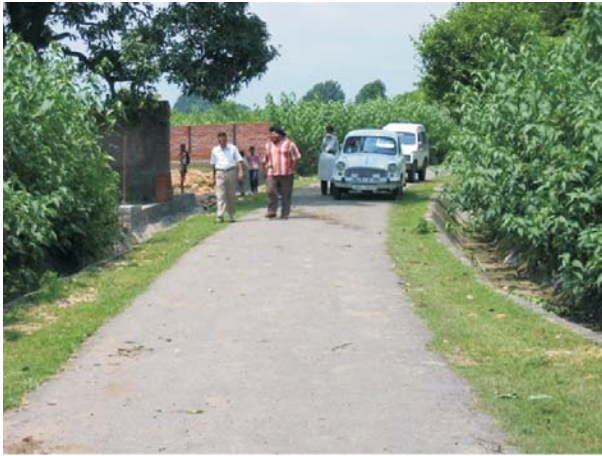
Road with side drains
