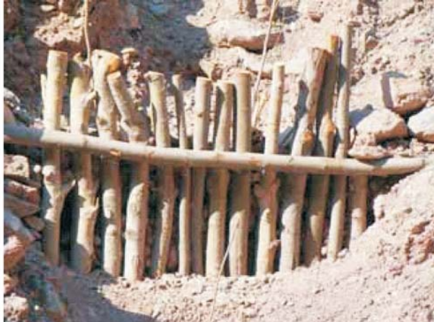
Newly constructed palisades
